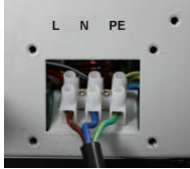
Fig. 8 AC terminals under AC terminals cover
